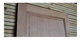
Detail of unpainted raised and fielded panel surface on ST102.
