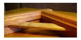
Detail of the moulding of Esstee door frames.
